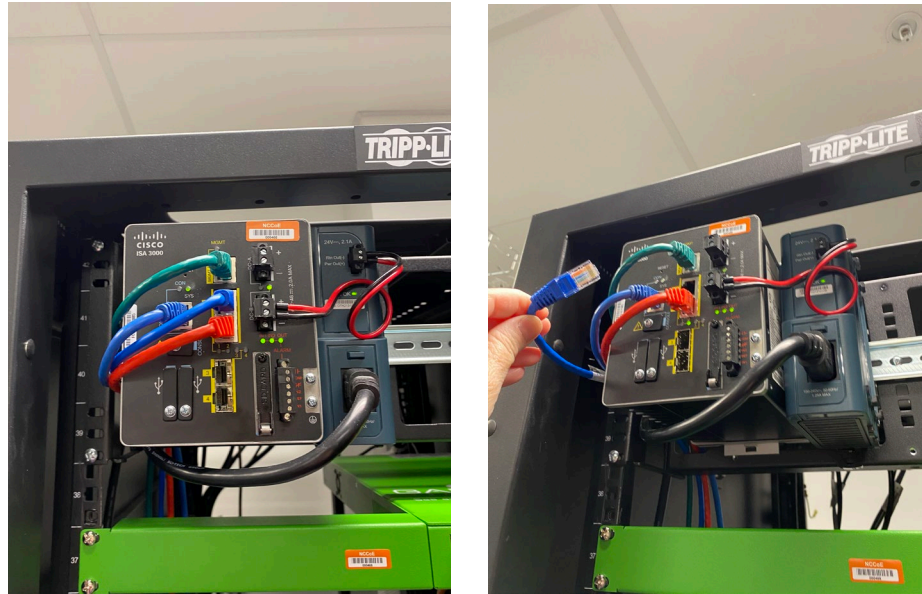
1746 Figure 4-41: Unplugging the Ethernet cable from the WAN port
